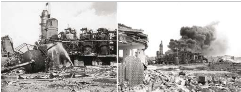
Fig. 4. The remains of the Nypro chemical plant at Flixborough after the massive vapour cloud explosion, June 1974 (CCPS 2005)
