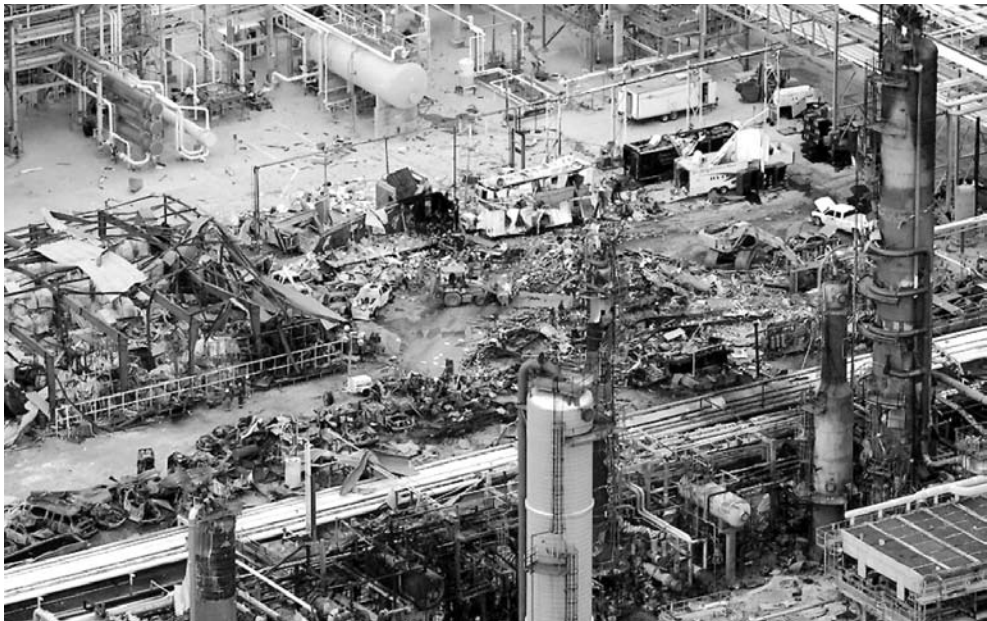
Fig. 2. Explosive damage to the building with portal steel frames (at the middle-left side of the picture; BP Texas City explosion March 2005) (CSHIB 2005)
