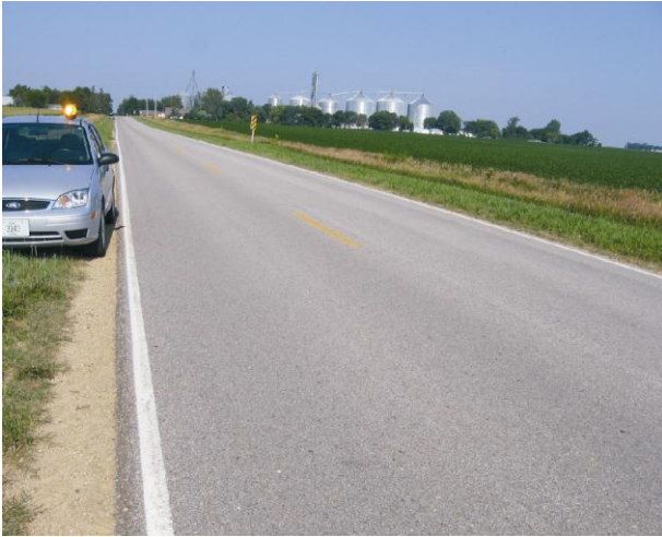
Fig. 7. Picture of distress-free AC surface on rubblized PCC layer (No. 1: C23 in Franklin County)
