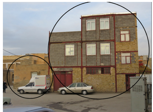
Figure 7. Two houses next to each others with significant different scales (Authors, 2018)
