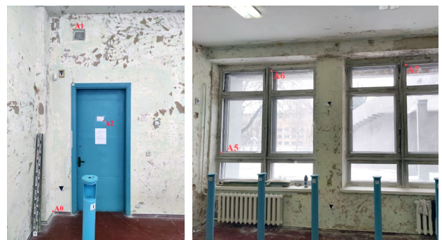
Figure 3. Example of characteristic points of room contours used for aligning the scanned point cloud
