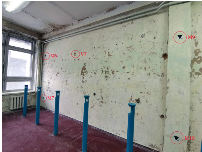
Figure 1. Fragment of the classroom wall with control markers
