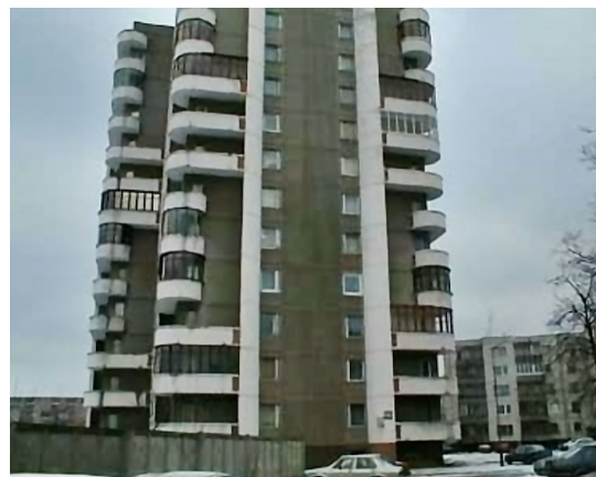
Fig. 2. Multi-storey building at Buivydiskiu st. 15, Vilnius
